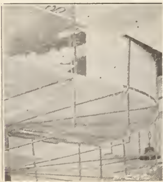
8. Another view of double duct construction around curves.
